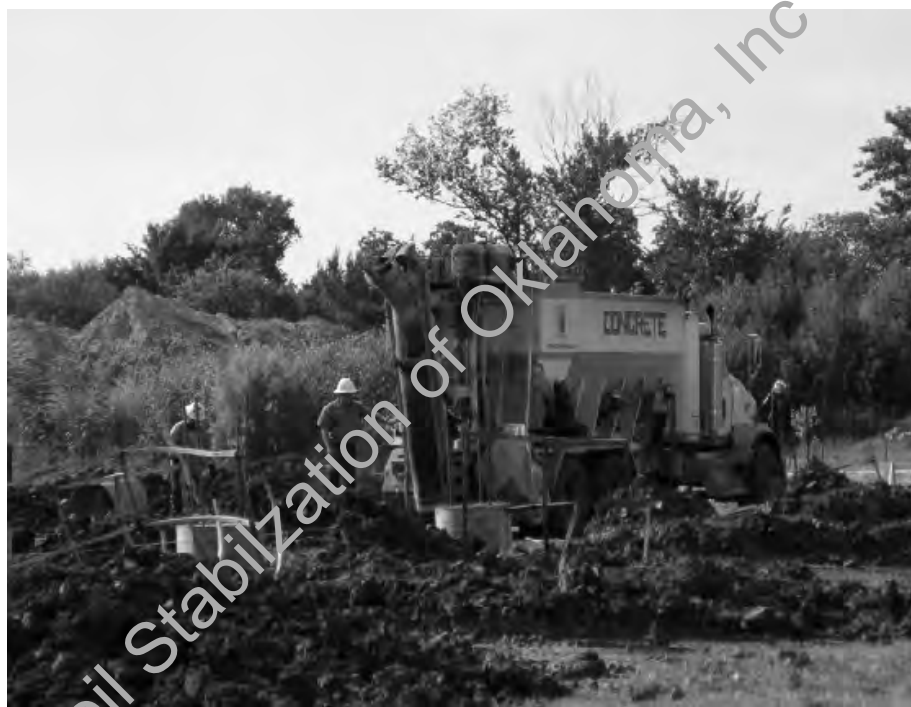
Figure 3.30- Pouring of Concrete Piers
