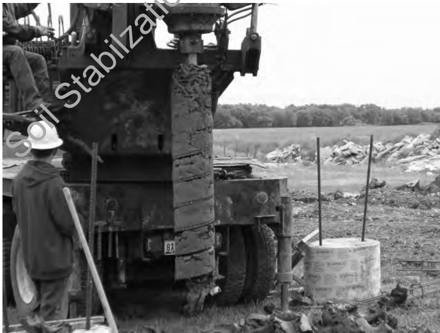
Figure 3.29- Drilled Shaft Installation
