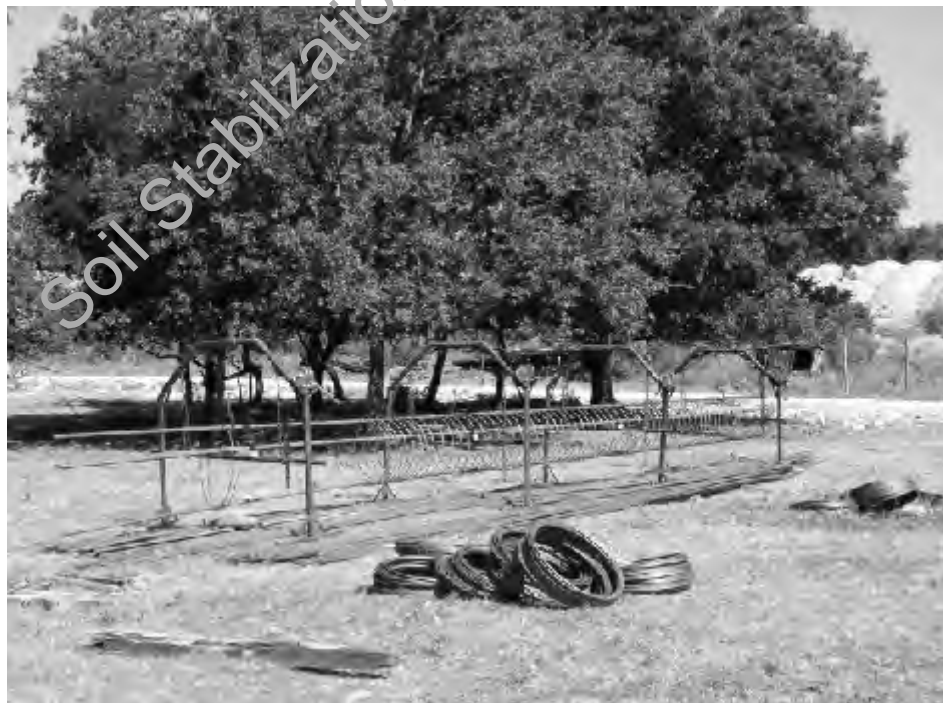
Figure 3.23- Reinforcement Cages Being Tied for Reaction Piers
