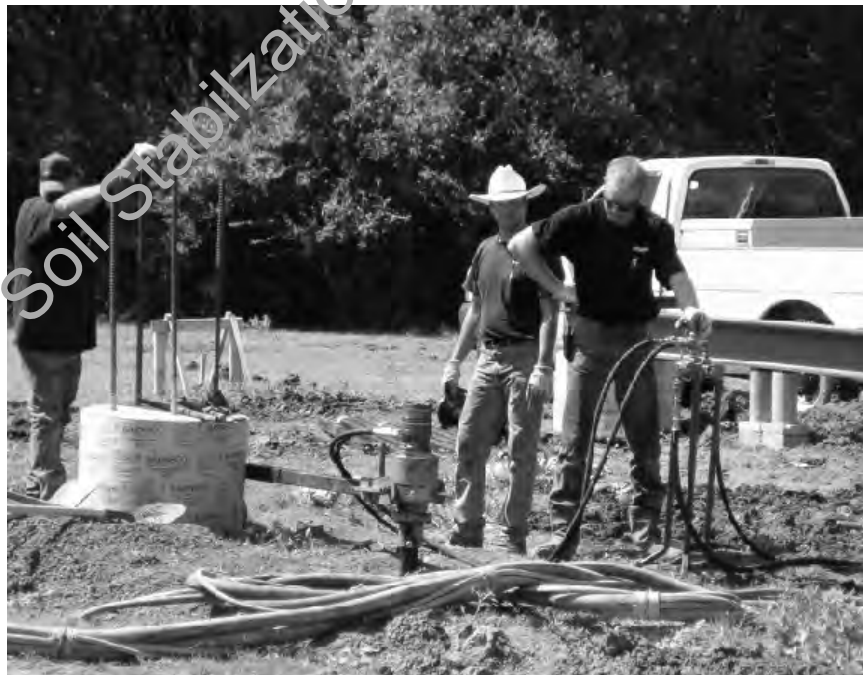
Figure 3.35- Installation of Helical Anchors
