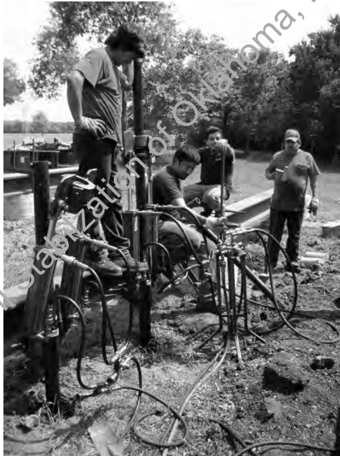
Figure 3.38- Installation of Pressed Steel Piles
