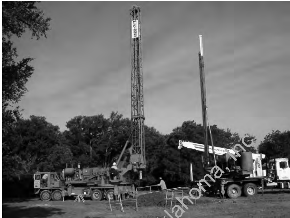
Figure 3.24- Installation of Reaction Piers
