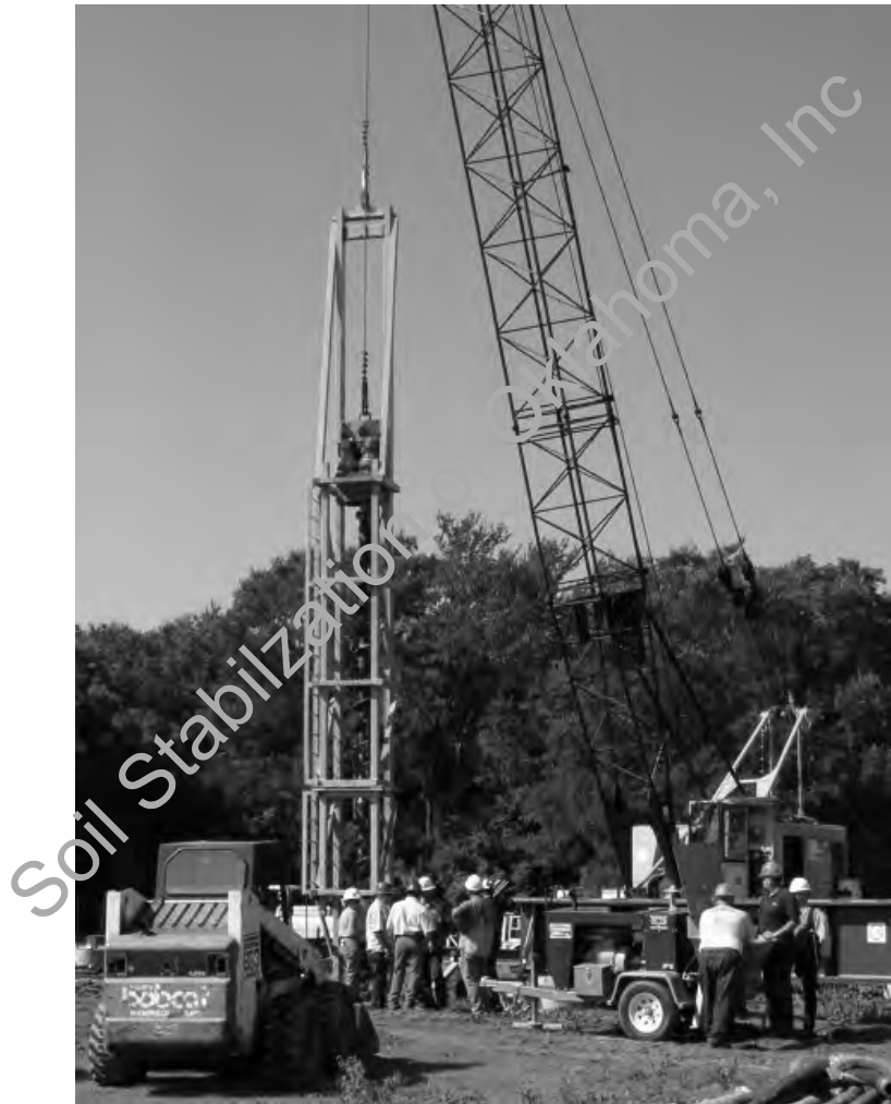
Figure 3.34- Installation of Augercast Piles
