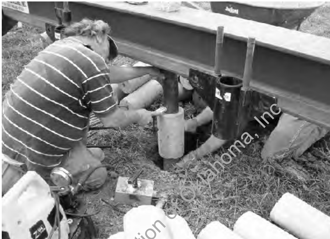
Figure 3.41- Installation of Pressed Concrete Piles
