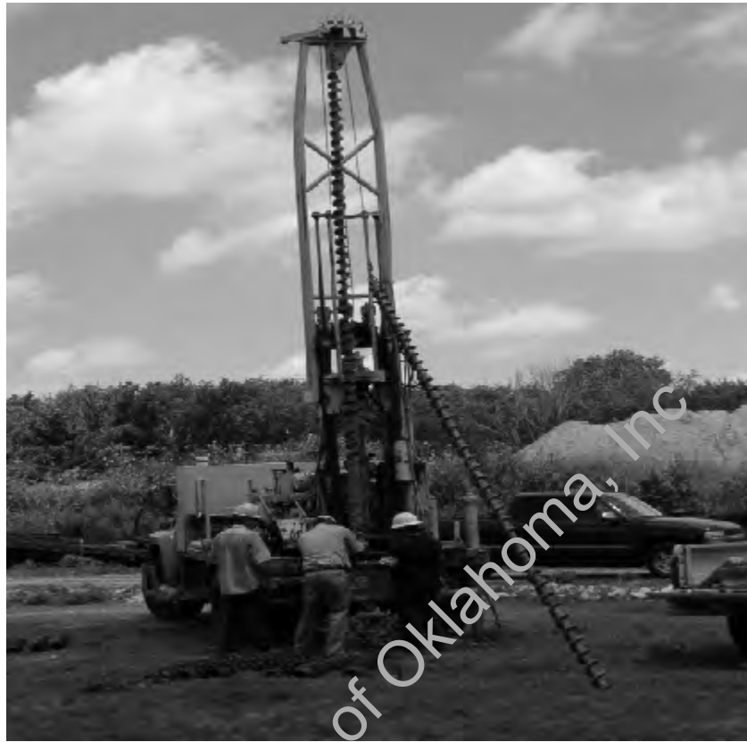
Figure 3.8 - Boring Operations Using Augering: Log #1
