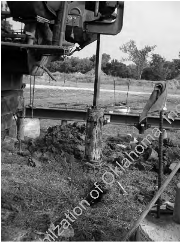
Figure 3.32- Installation of Belled Piers
