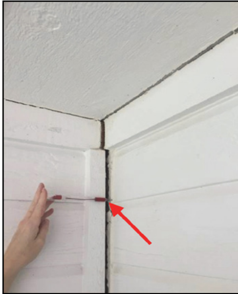
Figure 1-16. Siding separation.
