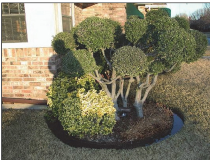
Figure 2-10. Do not excavate a border for flower beds next to houses to prevent ponding of water near the structure.
